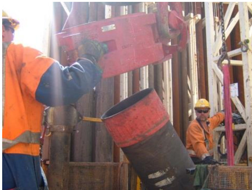
Ensure casing collar comes inside casing make up device
