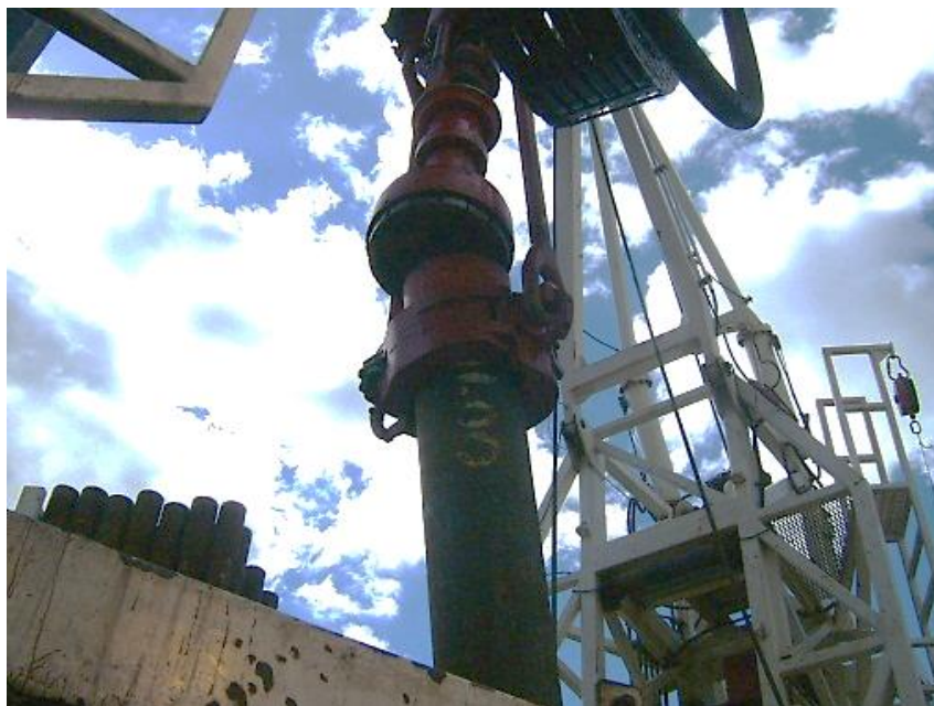
Lower casing into collar
