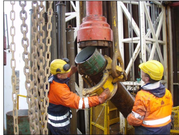
Casing brought up to drill-floor
