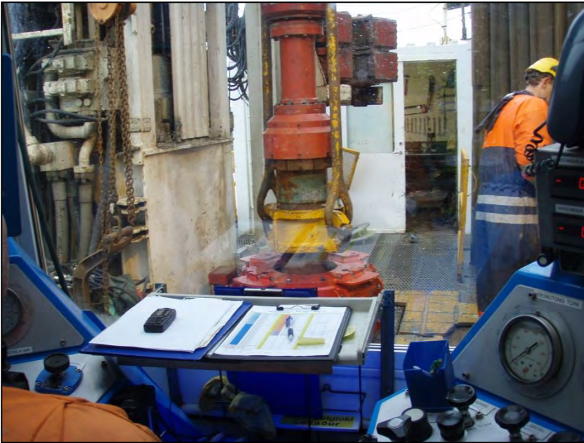
Casing lowered into casing slips
