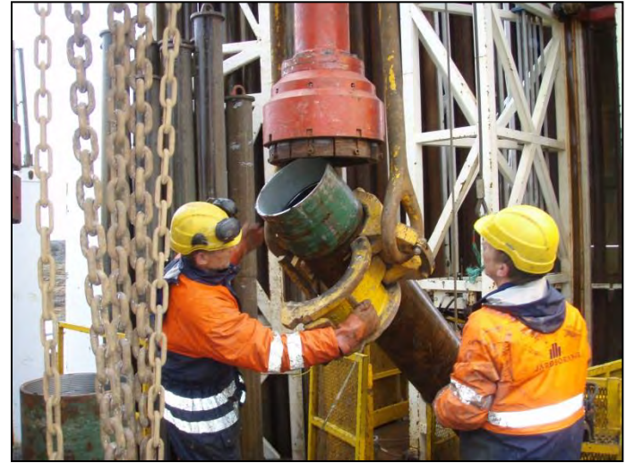
Casing brought up to drill-floor
