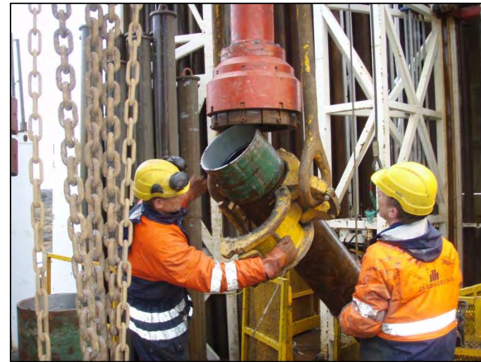
Casing brought up to drill-floor
